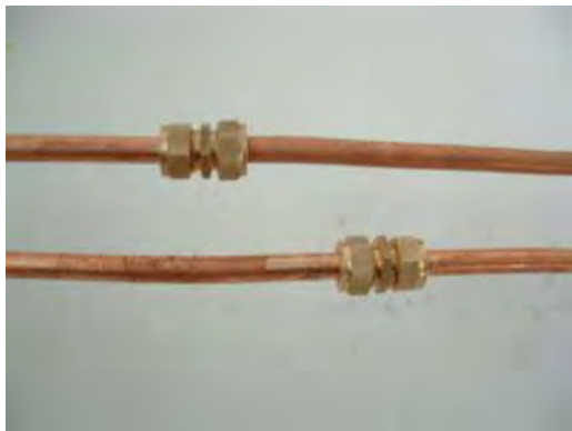
Figure 9: Joining copper pipe with unions.
