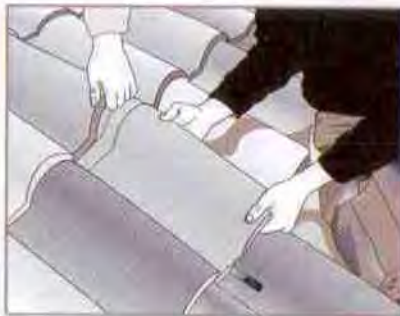
Figure 14: Installing collector straps to roof, steps 7-12
