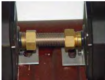
Figure 19: Two collector headers joined.
