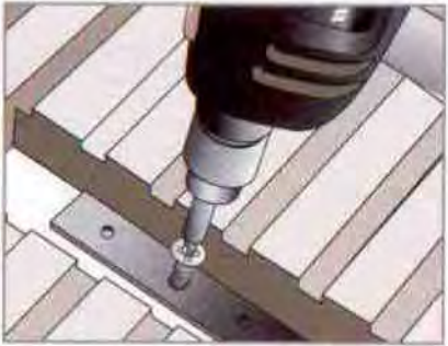
Figure 14: Installing collector straps to roof, steps 7-12
