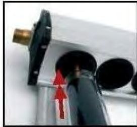
18. Push the vacuum tube to the manifold hole, make sure vacuum tube fix with the anti-dust circles tightly
