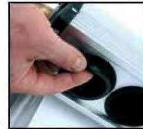
12. Turn solar collector back and install anti-dust circles
