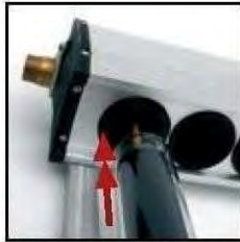
14. Push the vacuum tube to the manifold hole, make sure vacuum tube fix with the anti-dust circles tightly
