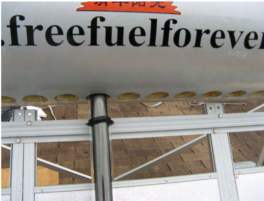
Figure 16: Tube inserted in tank.
