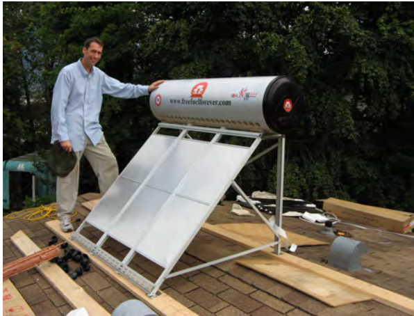
Figure 13: Level base for solar heater frame.
