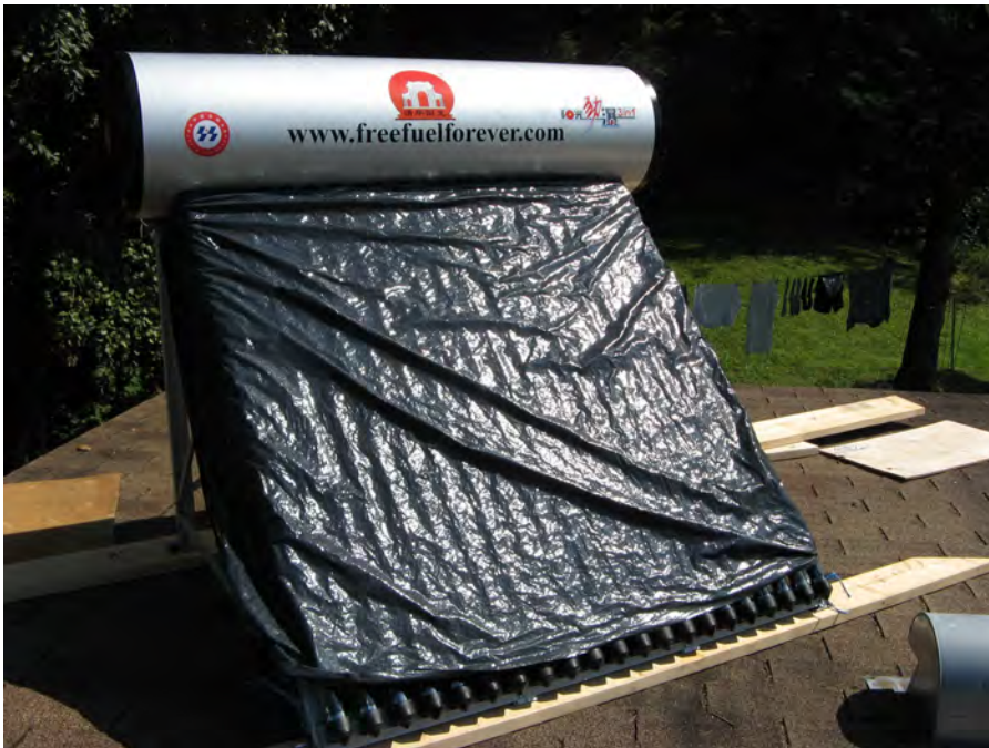
Figure 19: Complete solar heater covered to avoid overheat.
